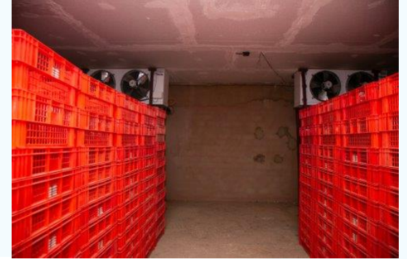
Cold store in an Adobe building
