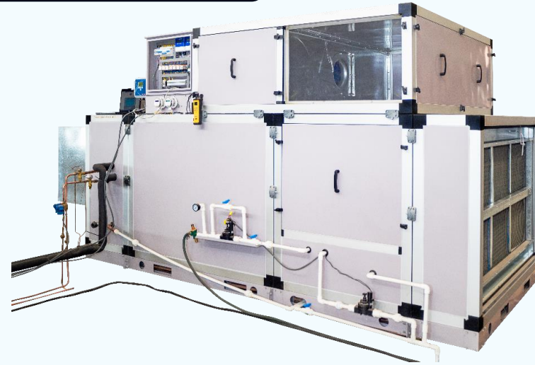
The HMX-DAMA integrated hybrid air handling unit (AHU) at the TECAM pilot site in Cali, Columbia.
